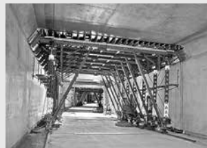
Tunnel Formwork
