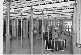
Slab Formwork
