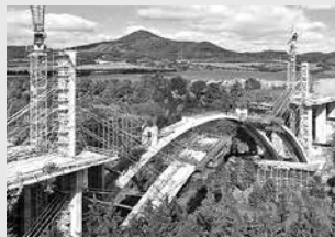
Bridge Formwork
