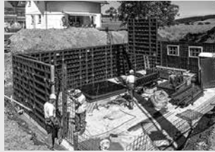
Wall Formwork
