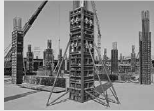
Column Formwork
