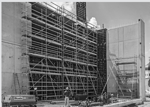
Working scaffolds construction
