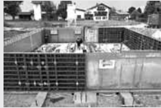
Wall Formwork
