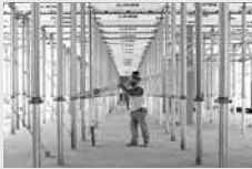
Slab Formwork
