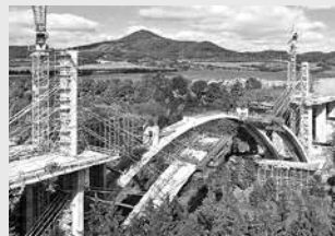
Bridge Formwork
