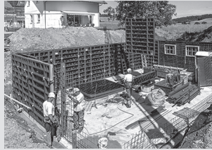
Wall formwork
