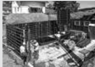
Wall Formwork
