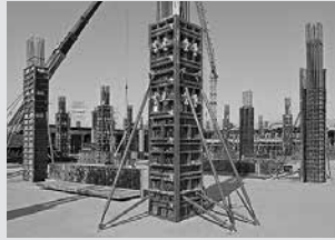
Column Formwork
