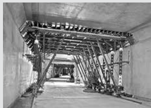
Tunnel Formwork
