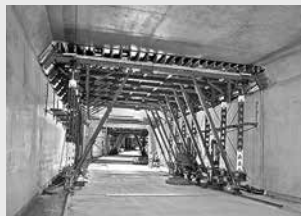
Tunnel Formwork
