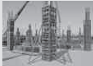
Column Formwork
