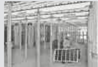
Slab Formwork
