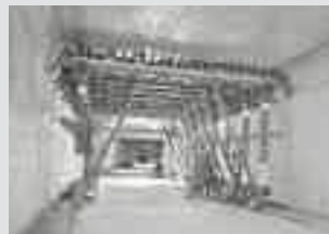
Tunnel Formwork
