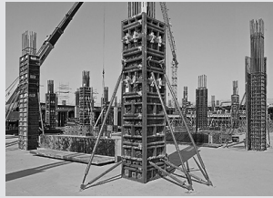
Column formwork
