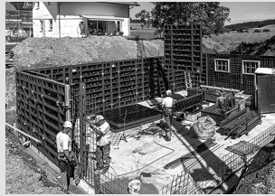
Wall formwork
