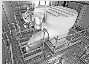
Working scaffolds industry
