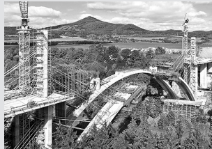
Bridge formwork
