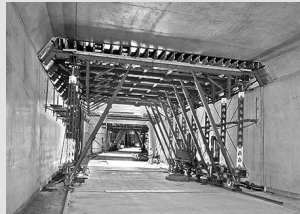
Tunnel formwork
