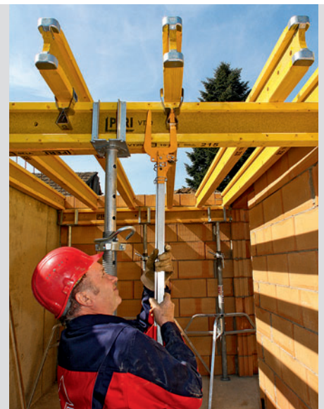
Using the same Fixing Tool, the Flexclips are also safely mounted from the ground.
