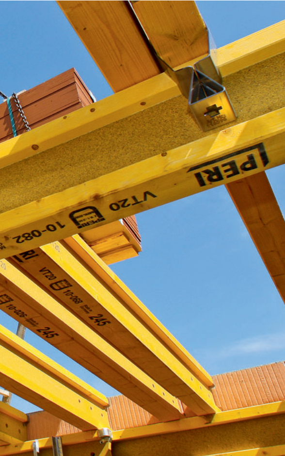
The PERI Flexclip secures the cross beams against tilting and is available in 3 versions, according to the girder combination.
