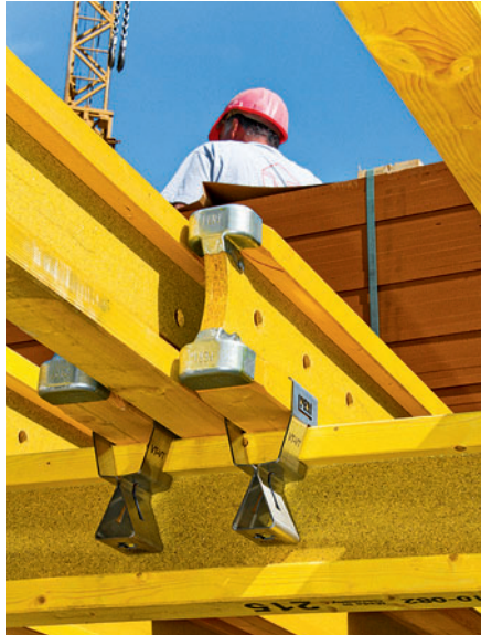
The PERI Flexclip secures the cross beams against tilting and is available in 3 versions, according to the girder combination.
