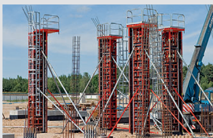
Coloum Formwork Systems
