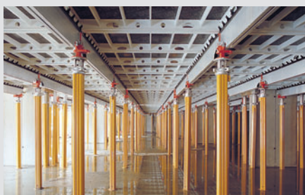
Slab Formwork Systems
