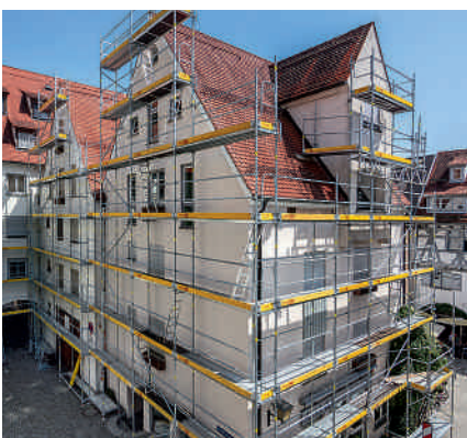
Renovation of an apartment building, Ulm, Germany
