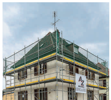
House renovation, Landau, Germany
