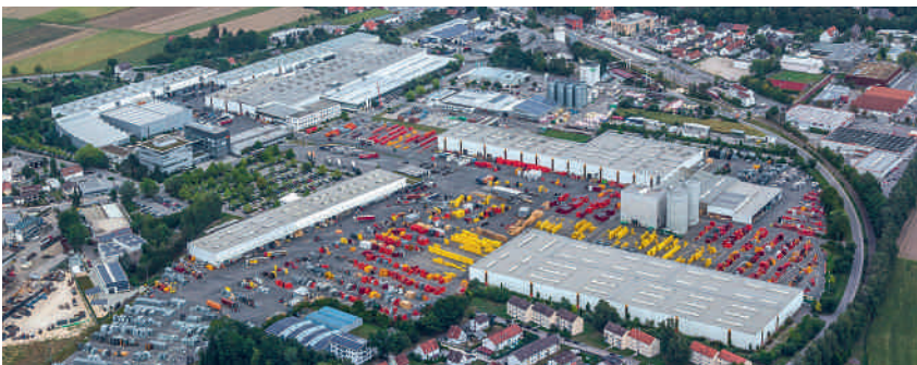
Since the company was founded in 1969, headquarters in Weissenhorn to the south of Ulm has been steadily expanded. The large majority of our PERI systems are still produced here today.
