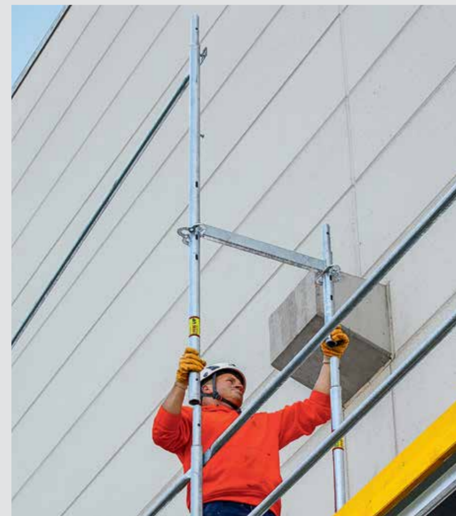
Faster assembly with lightweight individual components (e.g. brackets or frame components). Mounting takes place with virtually no couplers and a minimum use of tools.
