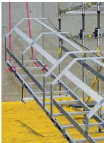
Pre-assembly of the ladder complete with ladder connections and ladder safety cage on the ground.
