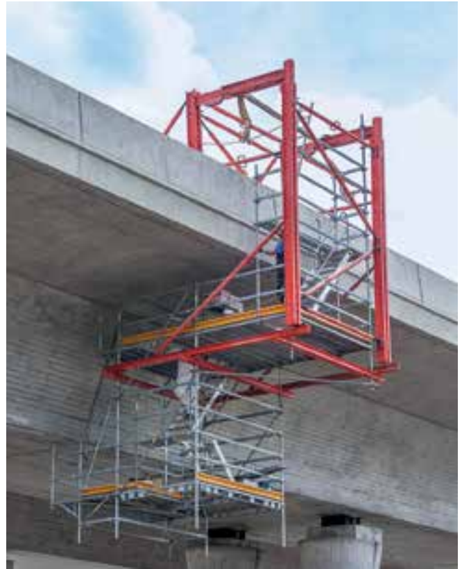
Due to site-compliant system combinations of the VARIOKIT Engineering Construction Kit and the PERI UP Flex Modular Scaffolding System, flexible and project-specific, optimized site solutions are possible.
